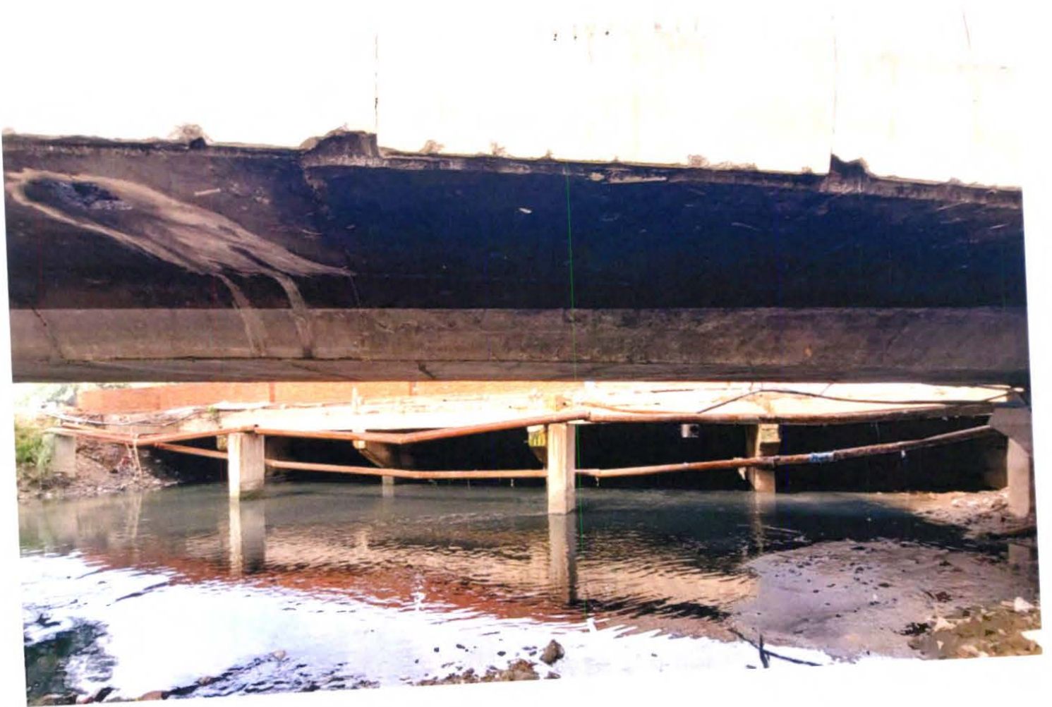
Sunehai Pulla Drain (Culvert)
